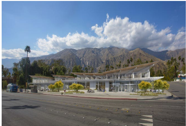
Aloe at Palm Canyon (under construction)
