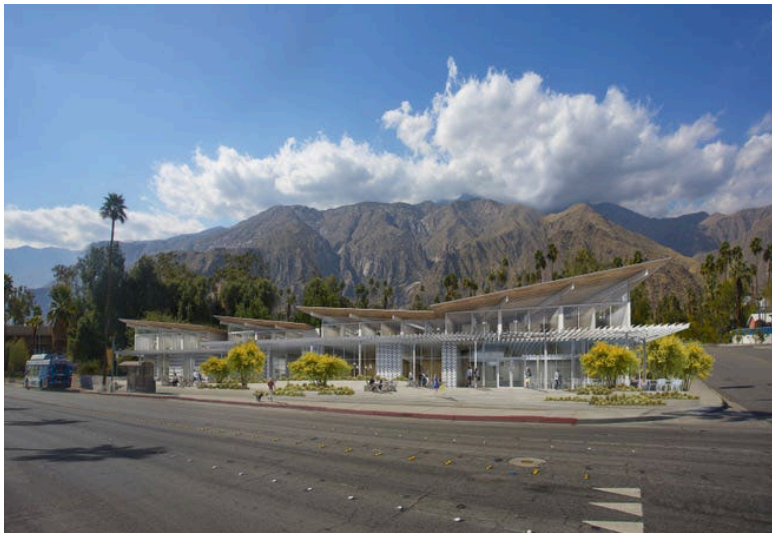
Aloe at Palm Canyon (under construction)
