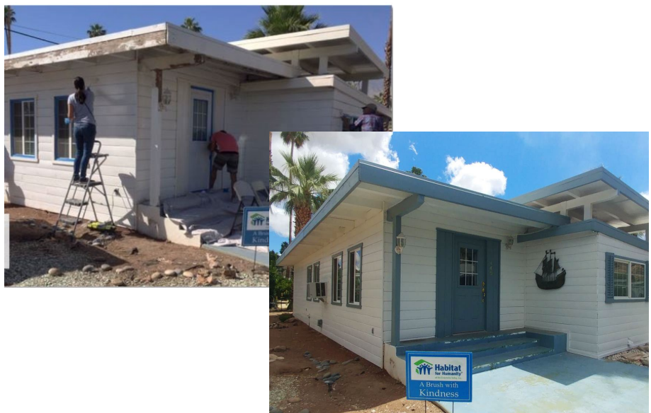
Habitat for Humanity housing rehabilitation projects.
