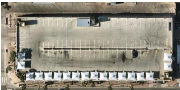
Overview of garage today
